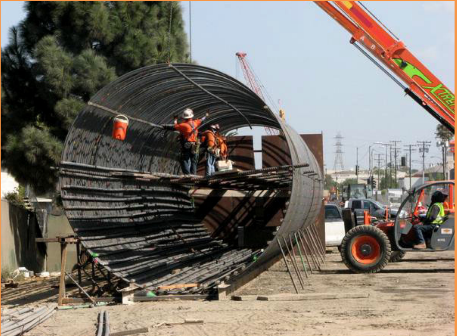
This is a giant column, tilted on its' side and being "tied down". The column coils are manufactured in a giant spool. The workers pull the spool open and tie long pieces of rebar to the spool to secure it in its' columnar shape. The workers are standing on rebar they've already placed and tied.
