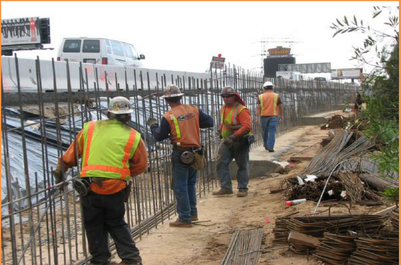
Four "big dumb white guys with pliers", placing 1/2" rebars every 8" or 16" (depending on the job). They're working on the 710 Freeway in Los Angeles. Looks easy, but 30 ft. straight up is the foreman yelling "next bar, move, Move, MOVE!". Notice the wire reels on the ironworkers' toolbelts, and the rusty stirrups for future work on the bottom right.
