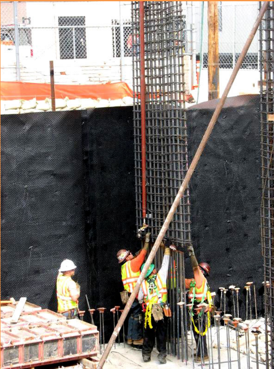
The vertical rebar in this column is usually more than an inch in diameter. This support column could be used for the foundation of a building, a parking lot, or whatever the blueprint specifies. We often were not told what kind of project we were working on - remember, we were just "big, dumb white guys"!
