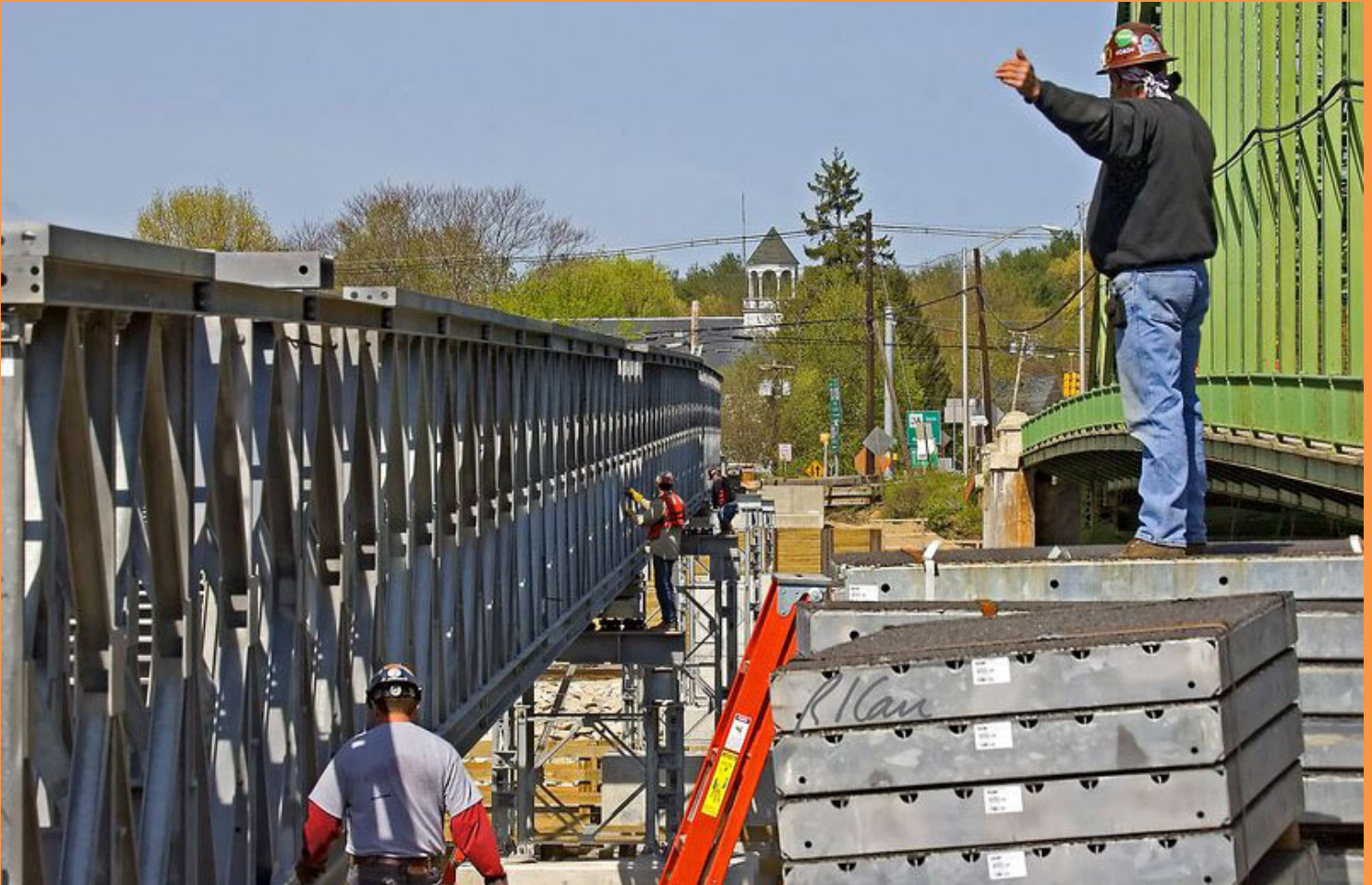
A bellowing foreman admonishing his crew: "Next bar...move – Move – MOVE!"
